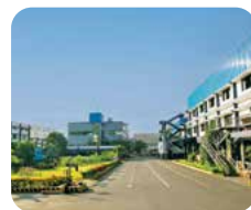
Igarashi Motors India Ltd, India
